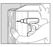
To ensure the filler piece stays in place, first fasten a support strip to the wall. Drill holes in the cabinet for the screws you'll use to fasten the cabinet and filler piece together. Put the filler piece into place. Put screws through the holes you have drilled. When all your filler pieces are in, caulk around each one with silicone for an airtight seal.
